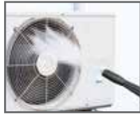
Aircor Condenser Cleaning
