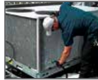
Aircor Condenser Cleaning
